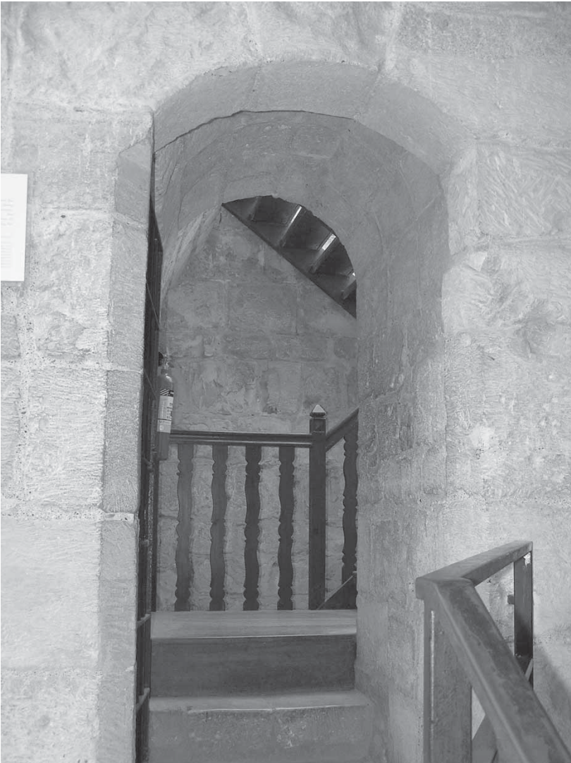
Fig. 35: Limassol Castle, upper level of cells, partly restored doorway in cell lodged in hall's southwestern angle [M. Olympios].
